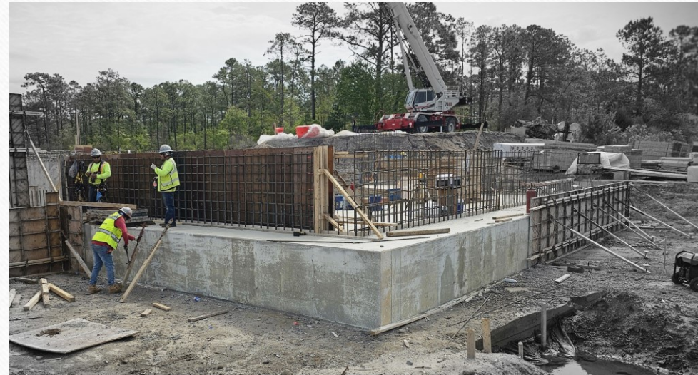
Tying Steel On The Upper Dam Spillway Inlet Weir
