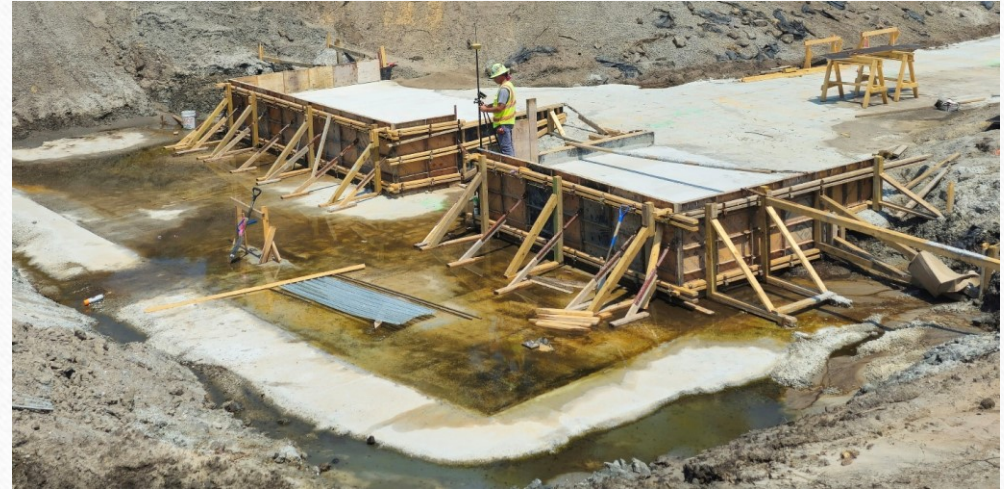
Surveyor Verifying Control Point on Pine Lake Dam
