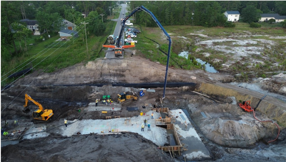
Pouring Pine Lake Dam Spillway Mud Mat
