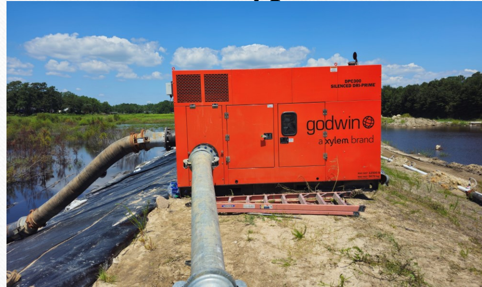
Mobilized 12" Pump at Sanford Dam Bypass Canal
