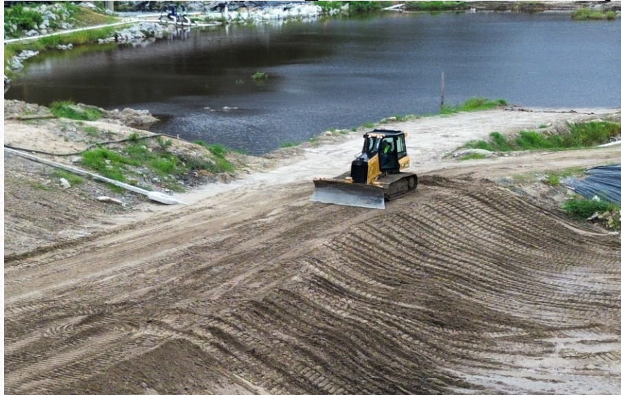
Repair Erosion Rills on Sanford Dam post TS Debby
