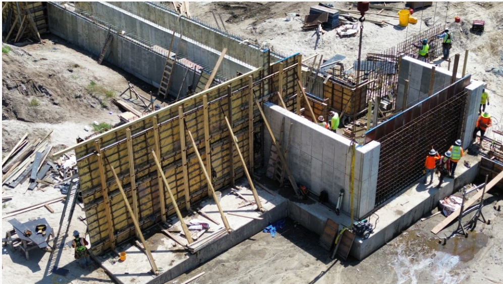
North Lake Spillway Inlet Steel & Form Work
