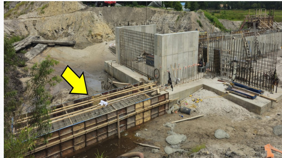
North Lake Dam Spillway Low Level Drain Form
